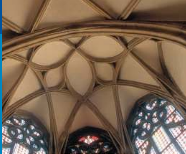
Late Gothic helical vaulted ceiling of the presbytery in the Town Hall chapel.
