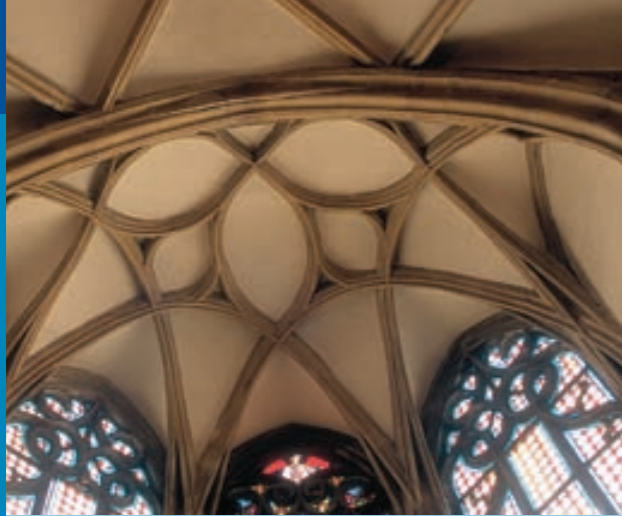
Late Gothic helical vaulted ceiling of the presbytery in the Town Hall chapel.
